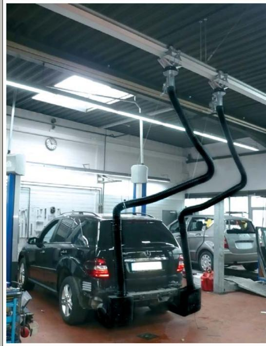
*2 SLS – Car systems running in a suction rail from type SSK 150 for cars with double-flow exhaust pipes at a Mercedes-Benz workshop*
