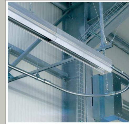
*Circuit gas extraction system for TÜV – car regular control stations.*
